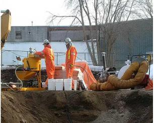
**Soil Stabilization (North Bay, ON)** Provided technical services to fill voids and stabilize soil underneath a footing during an expansion project at a waste treatment plant.
