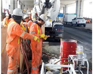
Chemical Grouting (Various locations, ON) Assisted an infrastructure contractor with a cellular grouting operation to backfill relined culverts along Highway 407.
