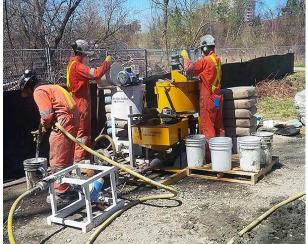
Water Cut-off (Markham, ON) Implemented a specialized leak sealing solution and customized grouting equipment for a municipal sewer rehabilitation project to repair leaks in a large-diameter sewer pipe.
