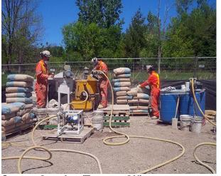
**Cement Grouting (Toronto, ON)** Performed microfine cement grouting and water stop operations using polyurethane resins. Provided sodium silicate grouting for soil stabilization in cross-passage tunnels in a light rail transit (LRT) line construction project.
