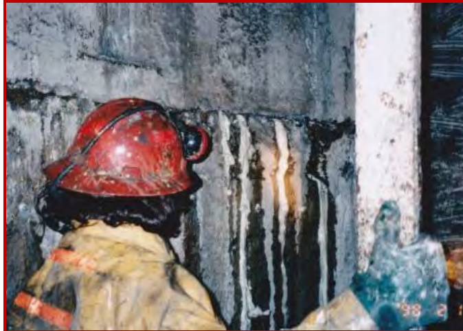
MME UNIVERSAL RESIN is used to stop water inflows through leaking concrete construction joints in an underground mine shaft.
