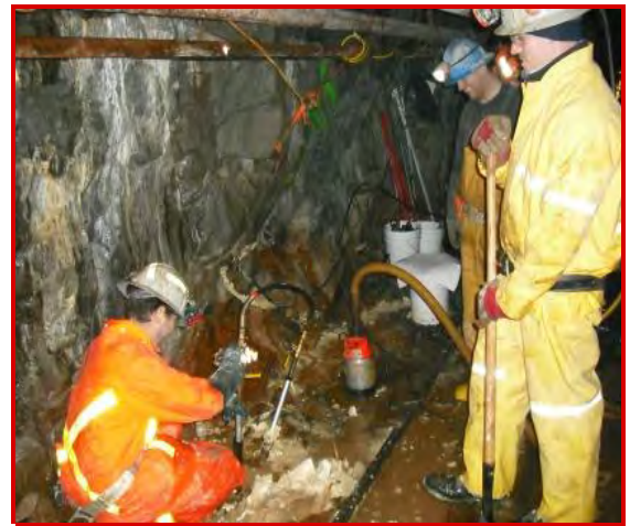
MME UNIVERSAL RESIN is used to stop water inflow problems for tunneling contractors.
