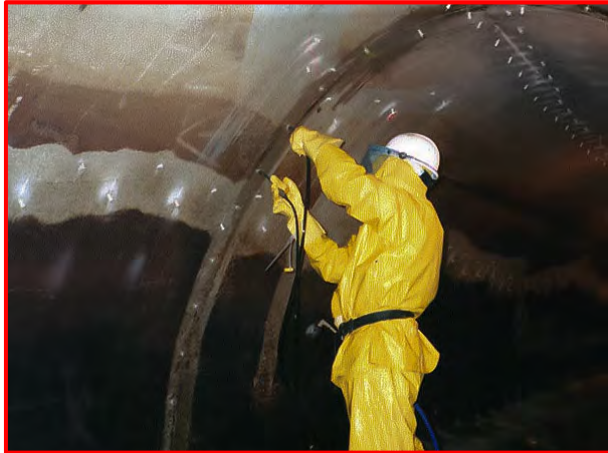
Cracks and construction joints in concrete structures are appropriately cleaned with CRACK FLUSHING AGENT prior to polyurethane injection.
