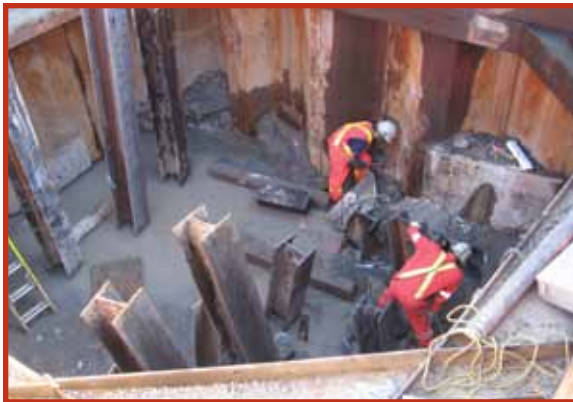
Heavy Civil, Water Cut-Off, Orangeville, Ontario A combination of cement grout and chemical grout is used to cut off large flows of soil and water in bridge construction.
