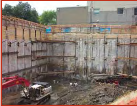
Deep Excavation, Cement Grouting, Toronto, Ontario Cement grout is routinely used to fill voids and seal water infiltrations in shored excavations.
