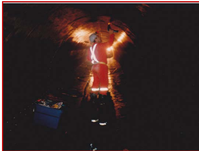
Cracks and construction joints in potable water structures are permanently sealed with MME FLEXIBLE RESIN.
