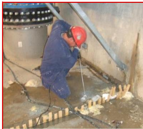
Leaking cracks are permanently repaired using MME FLEXIBLE RESIN.
