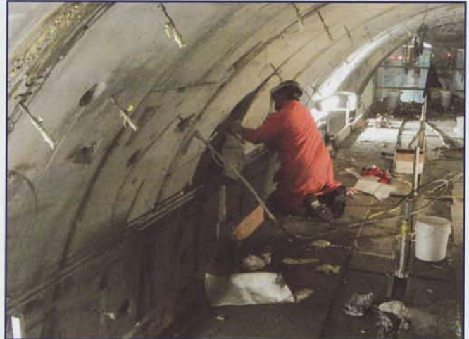
Multiurethanes Universal Resin is used to stabilize soil and cut off water flowing from leaking joints of precast tunnel segments.
