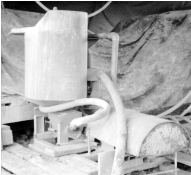
FIGURE 10 - COLLOIDAL GROUT MIXER
