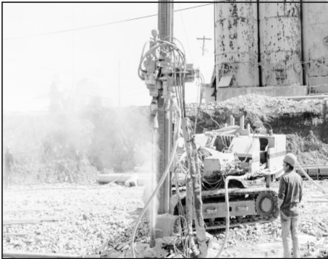
FIGURE 2 - DK 100 Drill Rig in Operation
