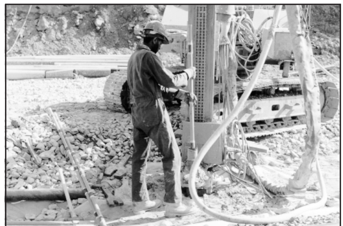
FIGURE 3 - Plastic Sleeve Pipes Being Installed
