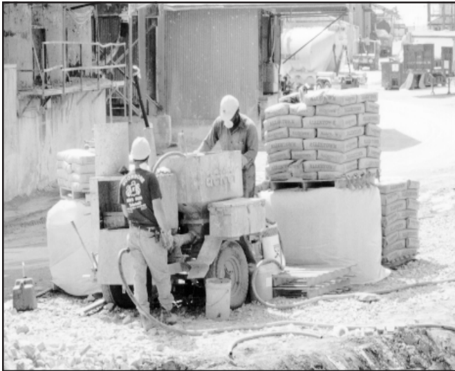
FIGURE 4 - Colloidal Grout Unit in Operation
