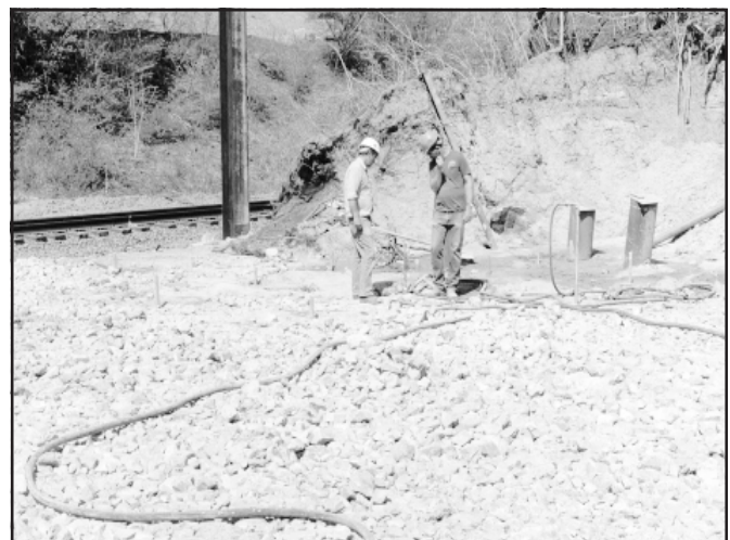
FIGURE 5 - Typical Sleeve Pipe grouting Operation
