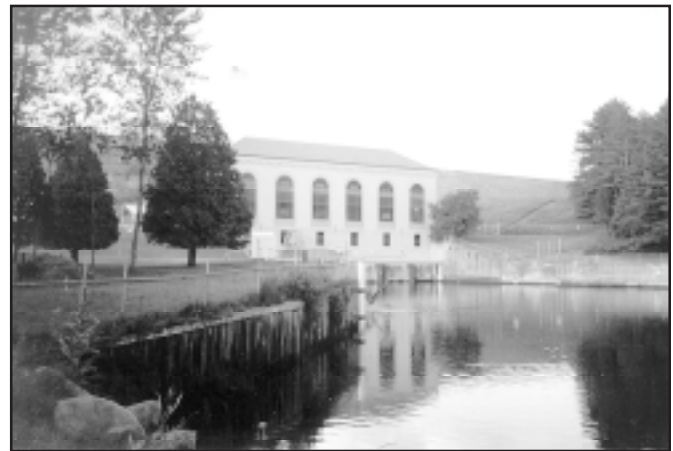
The tailrace of this hydro electric generating plant is typical of major project sites where MULTIURETHANES products are successfully applied without serious environmental consequences
