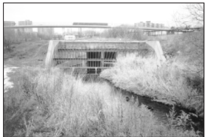
Storm sewer and diversion tunnel outfalls connecting directly with wetlands and fish spawning streams are sealed using MULTIURETHANES products to the satisfaction of local environmental authorities
