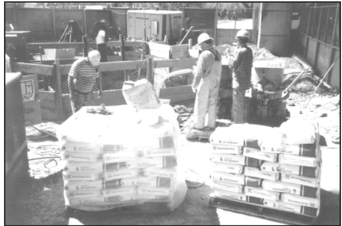
Cement grouting operation where colloidal mixers were used to prepare stable, balanced cement grout containing bentonite and superplasticizer additives for stabilizing loose, water-bearing soil adjacent to sheet pile wall surrounding vertical shaft; technical supervision by grouting specialist from MULTIURETHANES
